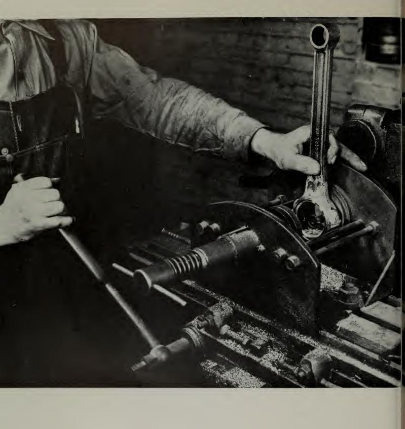
Approximately fifty per cent of the bearings have oil pockets which are cut by a hand milling machine as shown in the above picture.
